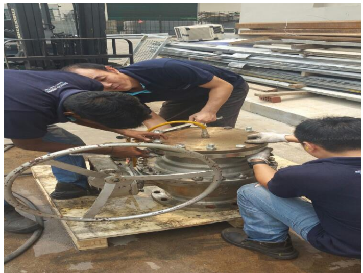
Valve and Pumps Servicing
