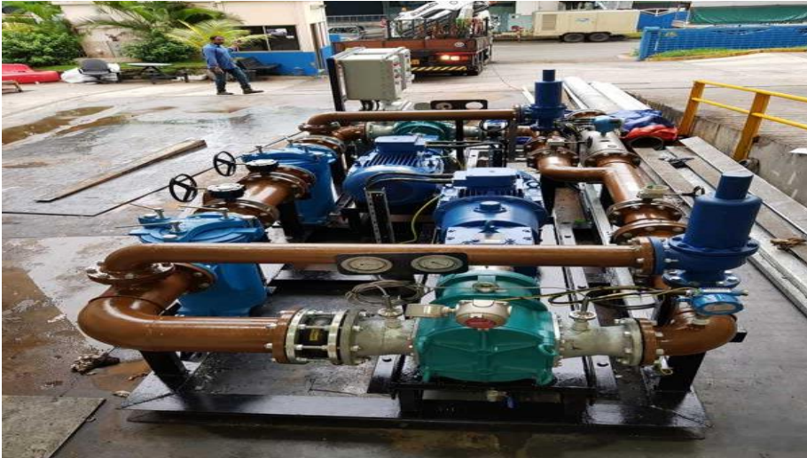
Fabrication of Pump Skids
