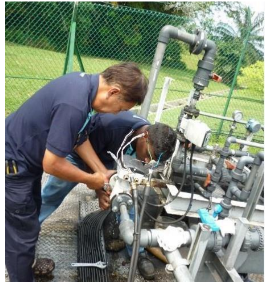
Installation and commissioning of flowmeters
